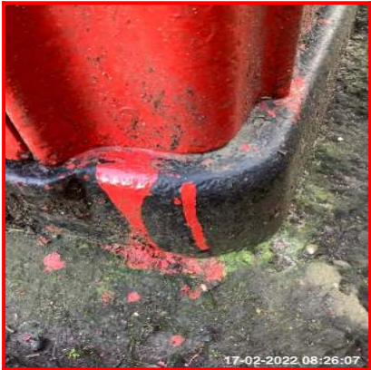
1.7.1 Exterior - Paint Splashes To Edges
