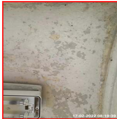
1.8.1 Paint Flaking To Interior
