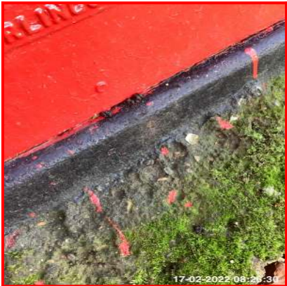
1.7.1 Exterior - Paint Splashes To Edges
