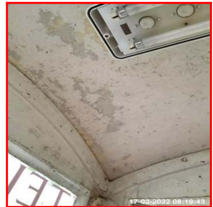
1.8.1 Paint Flaking To Interior
