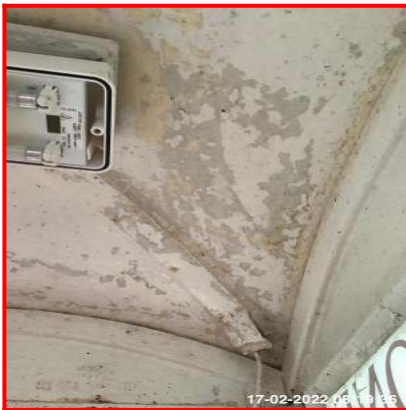
1.8.1 Paint Flaking To Interior
