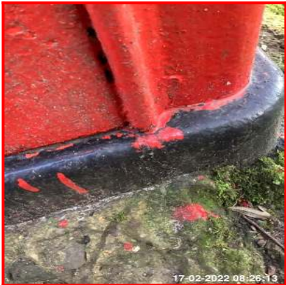
1.7.1 Exterior - Paint Splashes To Edges
