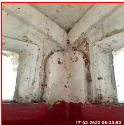
1.8.1 Paint Flaking To Interior
