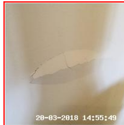
3.4.2 Cracking Behind Fireplace
