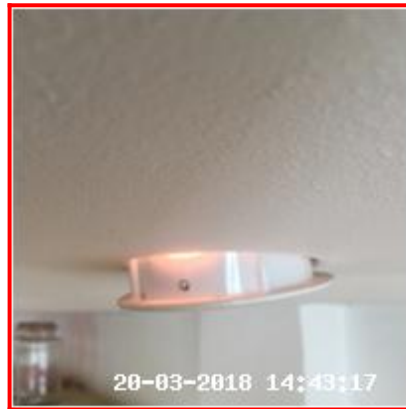
3.3.1 X2 Fitting Not Secure
