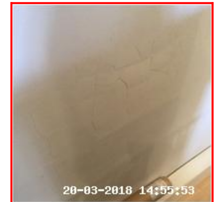
3.4.2 Cracking Behind Fireplace
