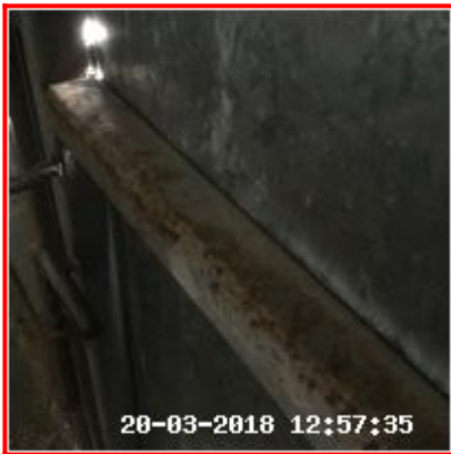
7.1.1 Surface Rust To Metal Frame 7.1.1 Surface Rust To Metal Frame
