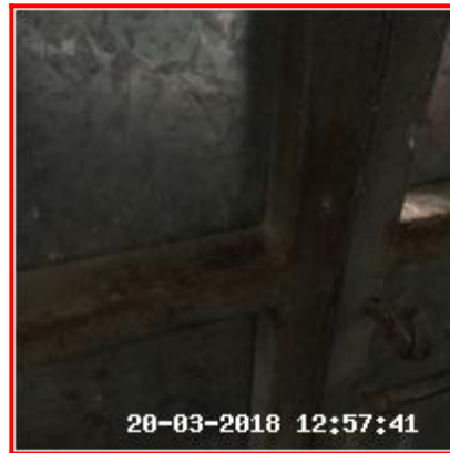
7.1.1 Surface Rust To Metal Frame 7.1.1 Surface Rust To Metal Frame
