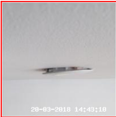
3.3.1 X2 Fitting Not Secure
