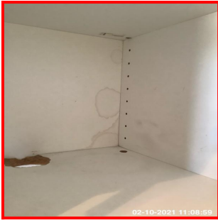
5.4.1 LHS Wall Unit Stained To Interior
