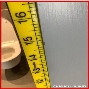
3.1.1 Chip To RHS Edge Above Lock Return
