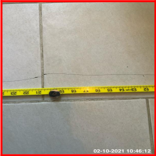
7.1.1 X2 Tiles Cracked By Door
