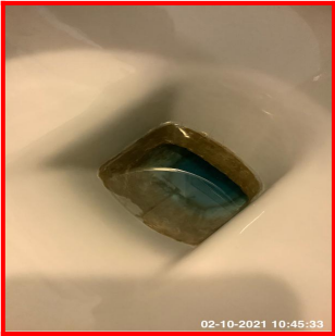
7.2.1 Discoloured Limescale To Throat
