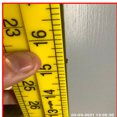
4.1.2 Small Paint Chip Above Lock Return
